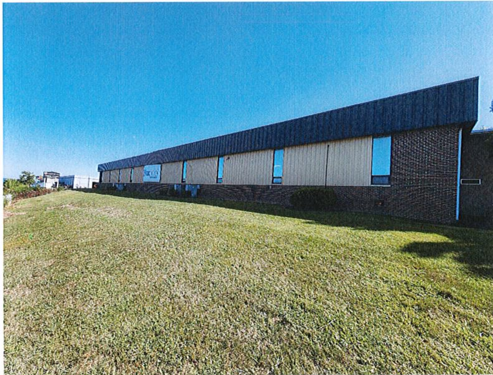
PHOTO 6 – Standing along I-83 right-of-way facing Northeast. Existing industrial building center of frame.
