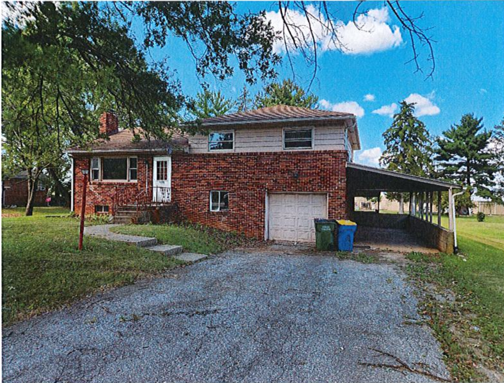
PHOTO 1 - Standing along Board Road facing West. Dwelling on proposed Lot #3.
