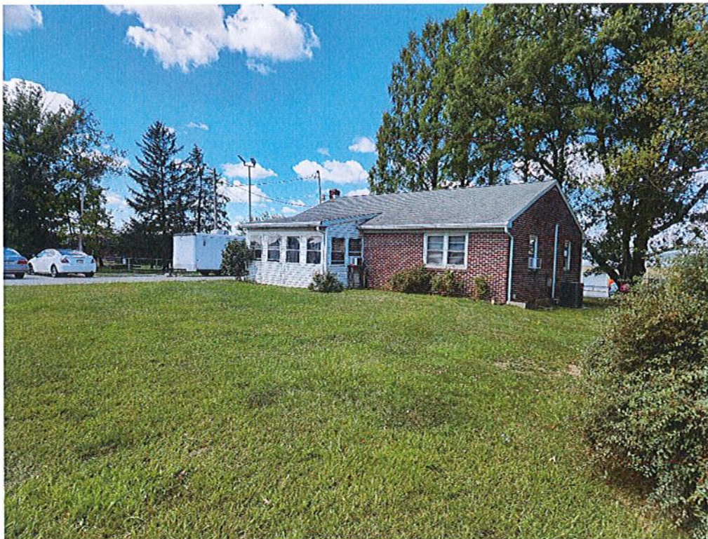
PHOTO 2 - Standing along Board Road facing West. Dwelling on proposed Lot #2.
