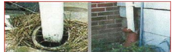
Downspouts that look like this could be connected to the sanitary sewer system.
